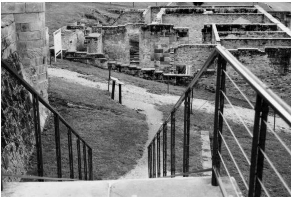
Law Courts from Guard Tower Steps
