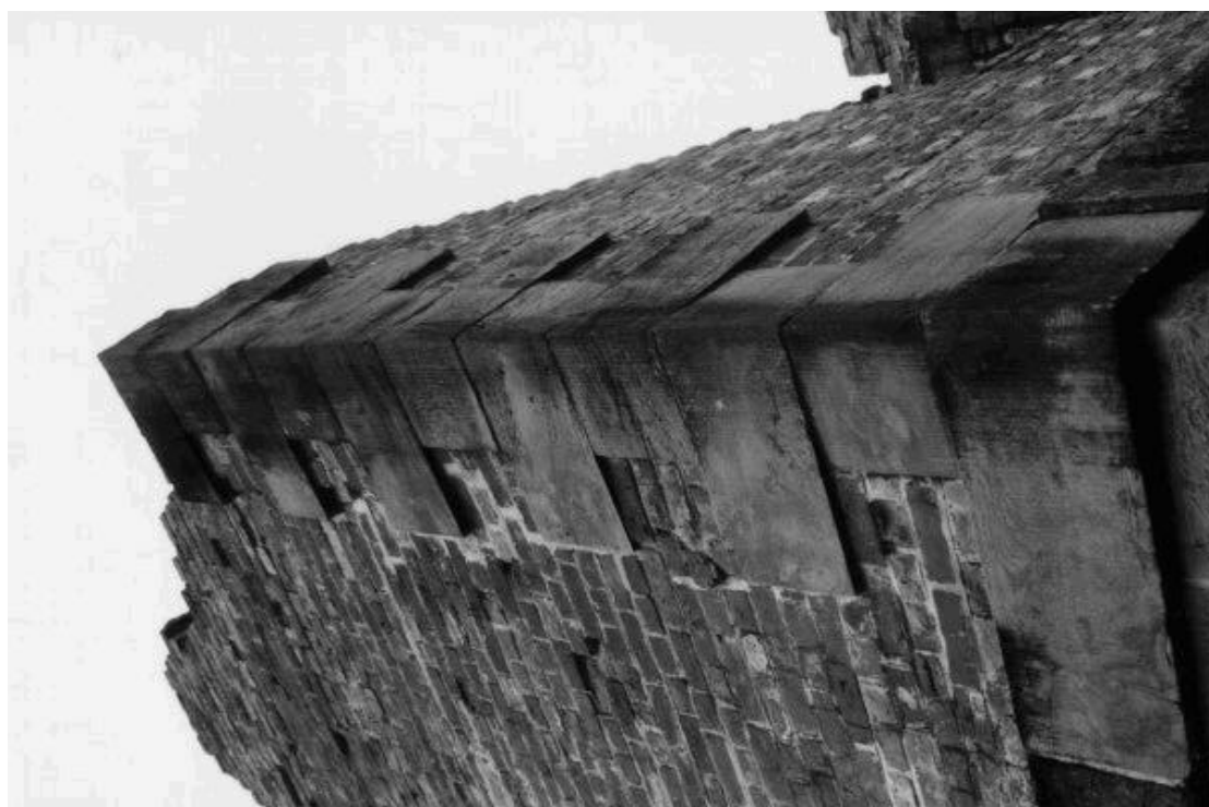
Hospital - South Western Corner
